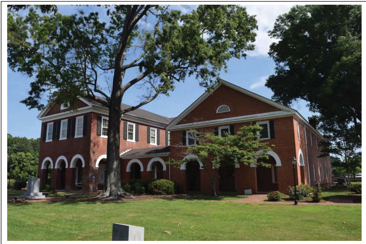
View to north. County courthouse, built 1849, at left; annex, built 1965, at right. June 1, 2022. R. Jacoby
