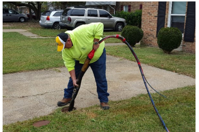
Arcadis conducted grouting work at Sullivan's Island, Aiken and HRSD VB340.
