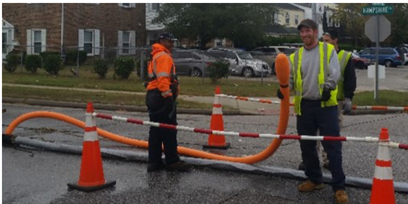
Arcadis conducted grouting work at Sullivan’s Island, Aiken and HRSD VB340.
