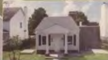
Designed as the "neighborhood's neighbor," the pump station blends seamlessly within the community.
