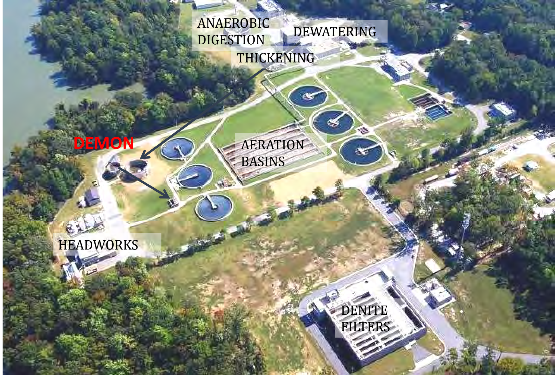
DEMON ® PNA at HRSD York River (15 MGD) - 2012
