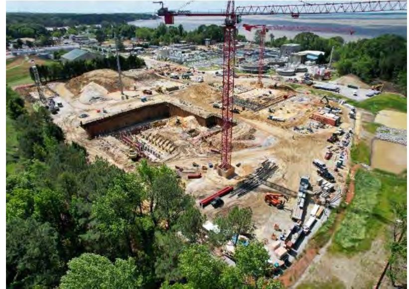
SWIFT Facility with Two Tower Cranes
