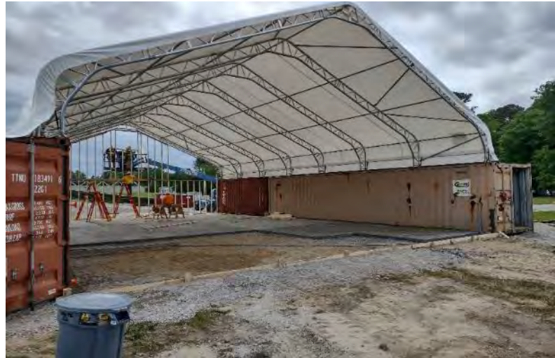
Contractors Temporary Field Shop
