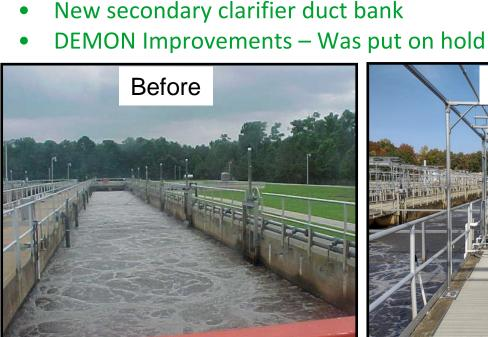
Baffle walls and big bubble mixing system
