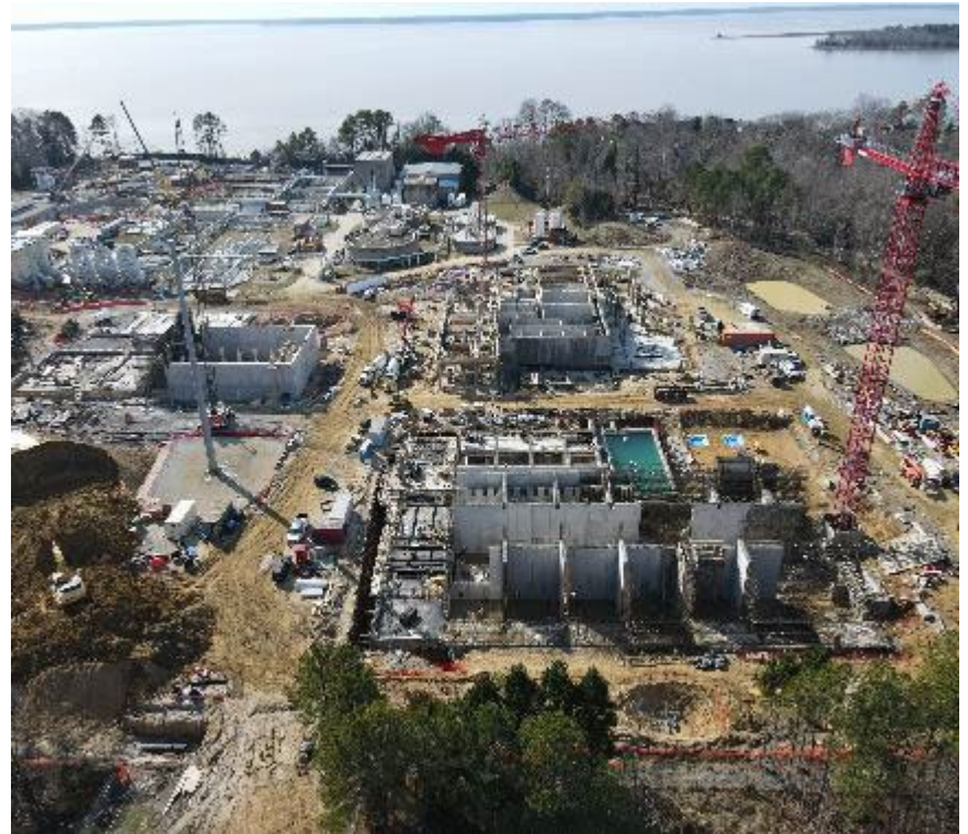
Aerial View of Construction
