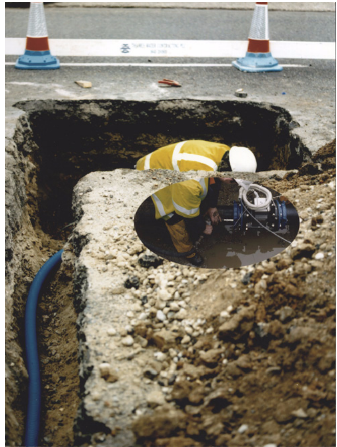
Underground Installation of MagMaster
