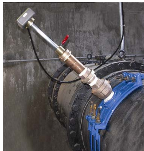
The ADFM Hot Tap sensor installs through a standard two-inch tap.
