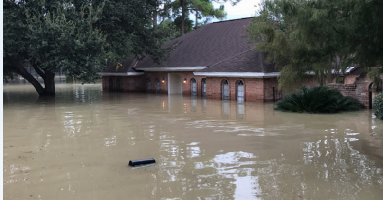
Flooding in Houston from Hurricane Harvey in 2017.
