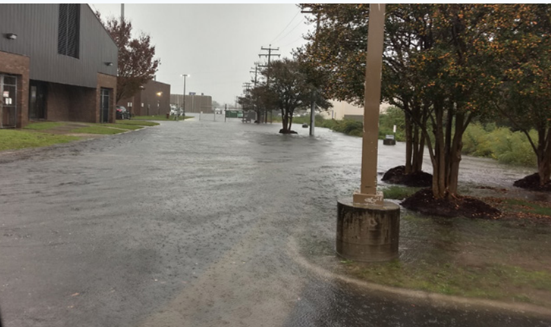
Example of rainfall runoff flooding – photo from the South Shore Administration Building on November 12, 2020.
