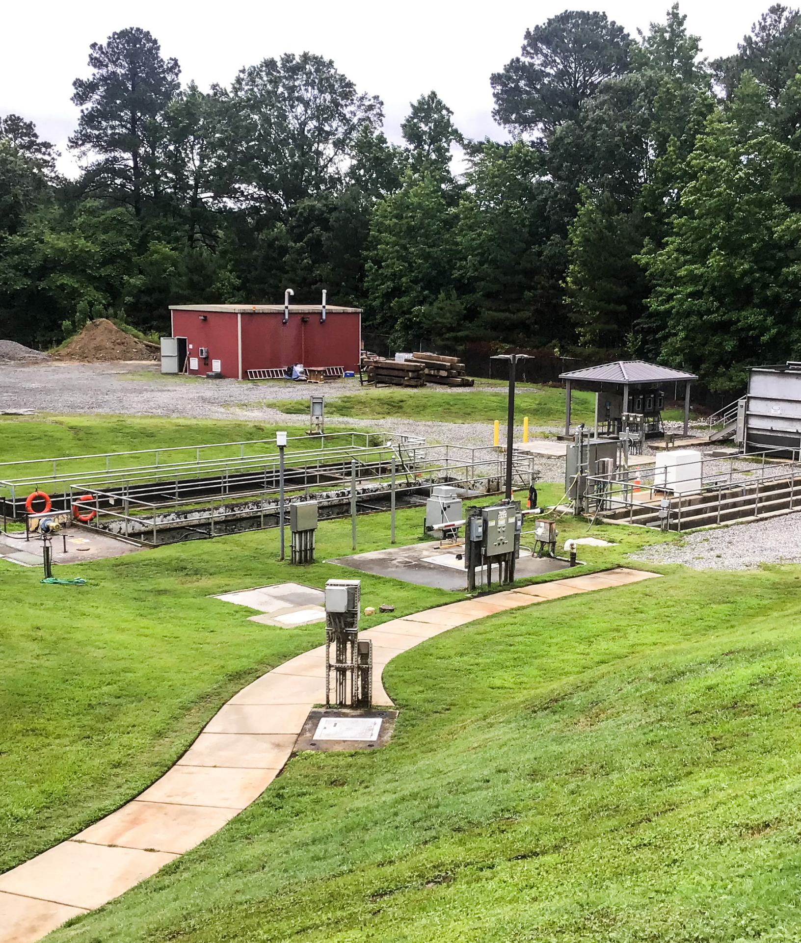
West Point Treatment Plant.
