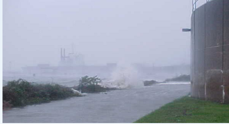
Example of storm surge flooding – photo from the Boat Harbor Treatment Plant during Hurricane Isabel in September 2003.
