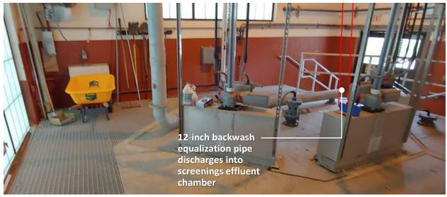
Figure 3-8: Pipe routing to the screenings effluent chamber
