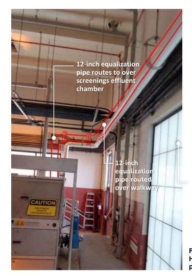
Figure 3-7: Entrance to Headworks Building and pipe routing
