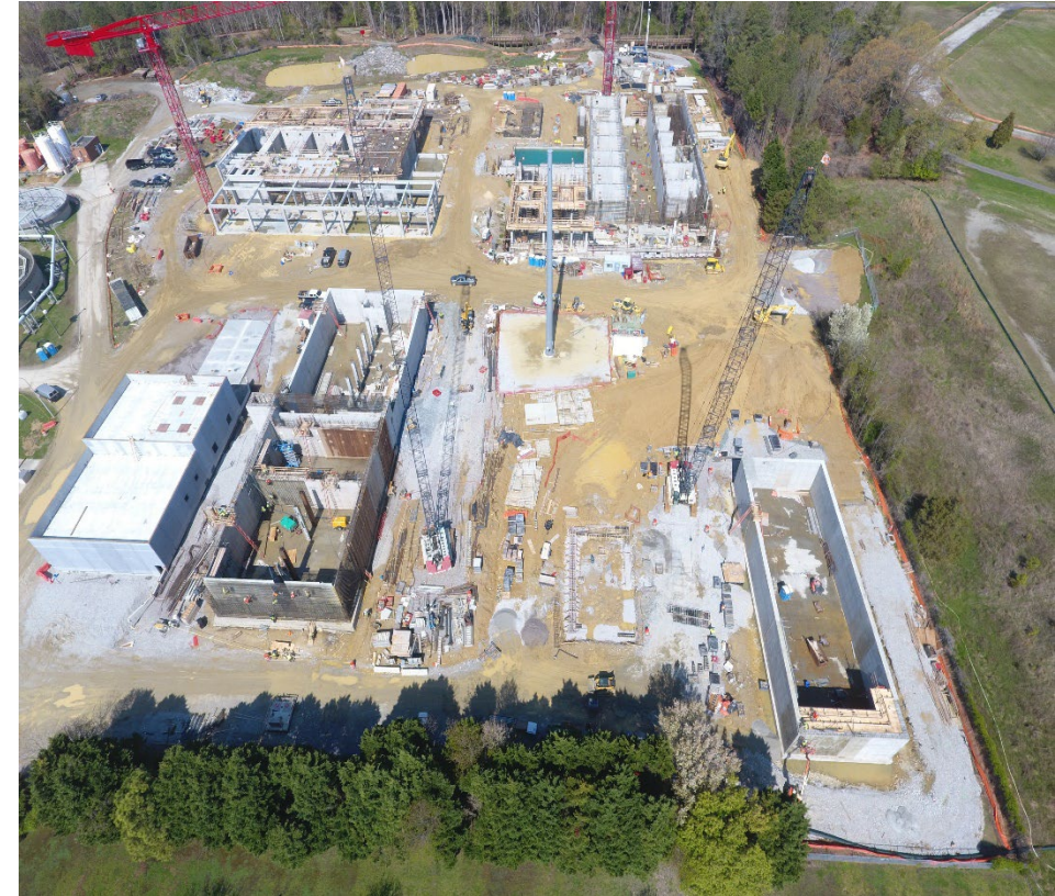
Aerial View of SWIFT Construction
