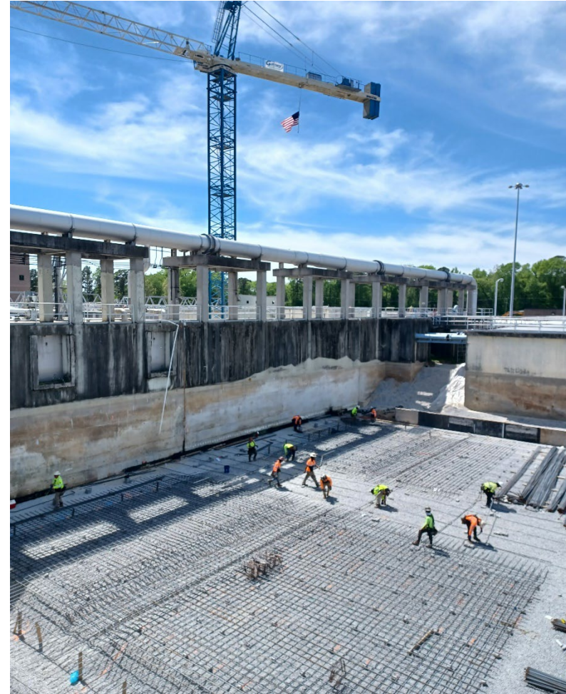
Installing reinforcing steel at Aeration Tanks 8 & 9.
