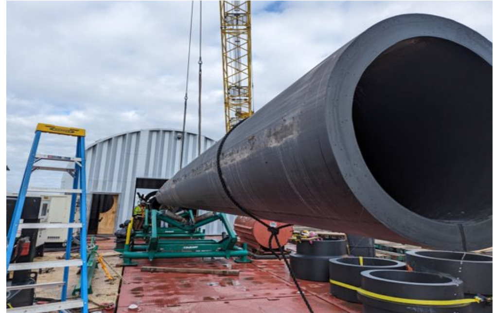
HDPE Pipe Fusing Operations
