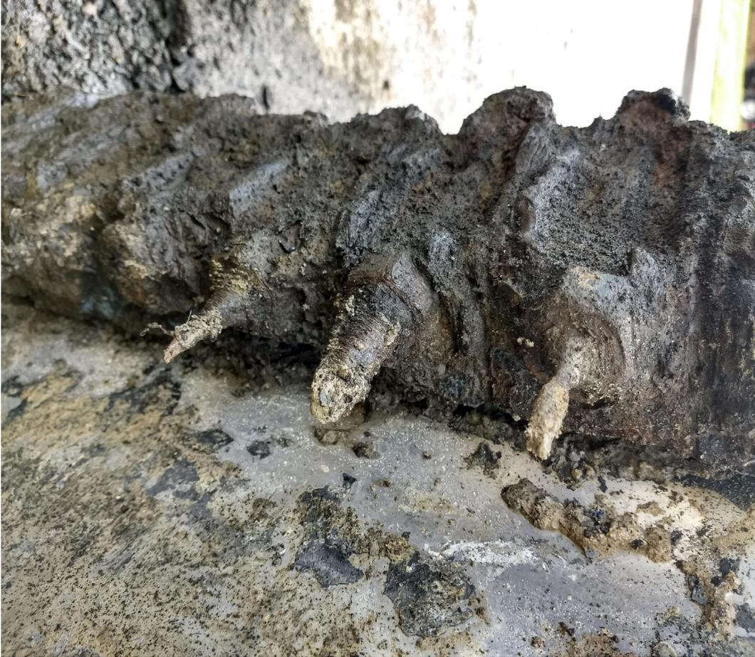
Corroded Bolts on Repair Clamp - Little Neck Road
