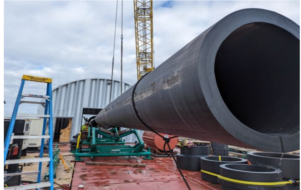
HDPE Pipe Fusing Operations
