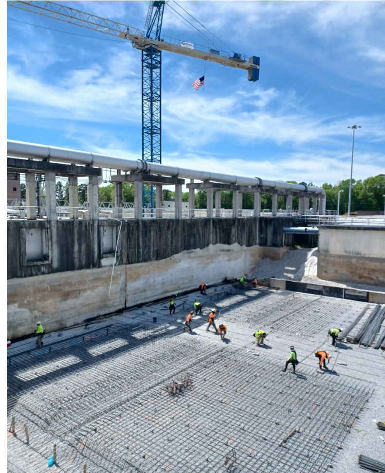
Installing reinforcing steel at Aeration Tanks 8 & 9.
