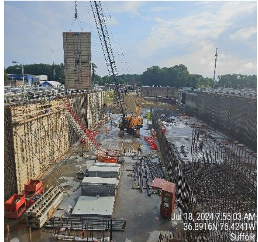
Installing wall forms at Aeration Tanks 8 & 9.
