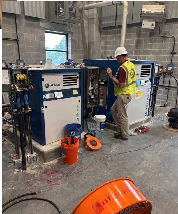
Blowers located in the Pre-Dewatering Building
