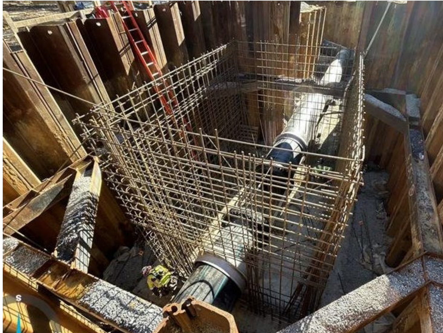
Instrumentation vault concrete
