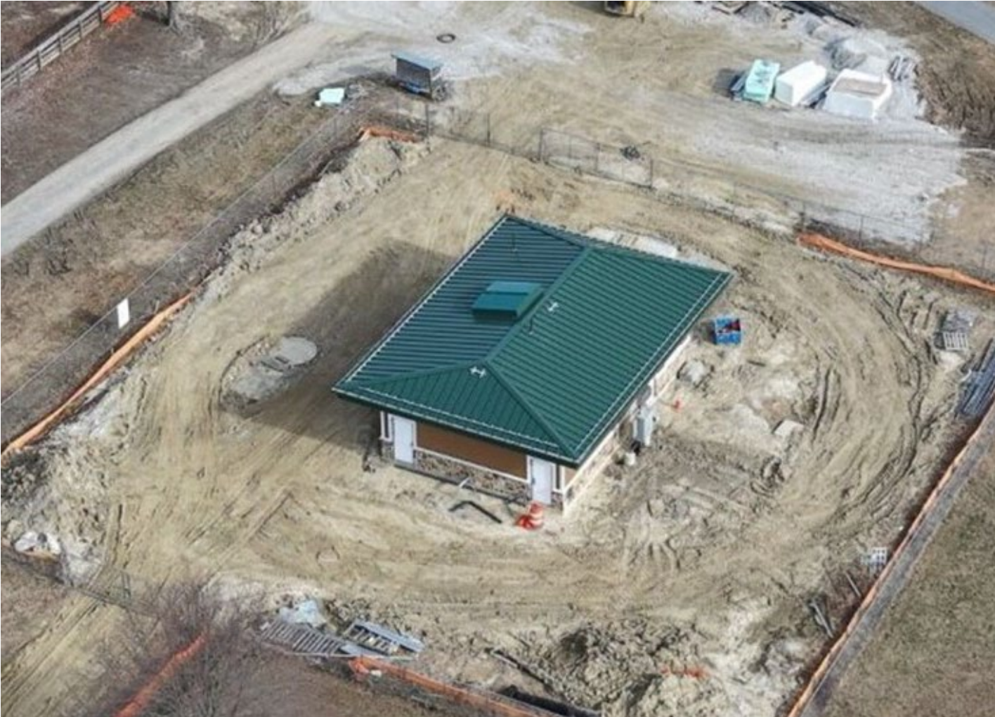
Installation of HVAC, plumbing and electrical systems at MAR Wells 1-4 and 7-10
