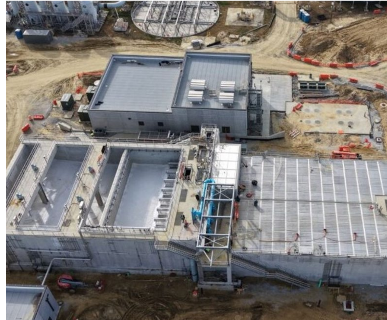
Installation and wet testing of MBBR media
