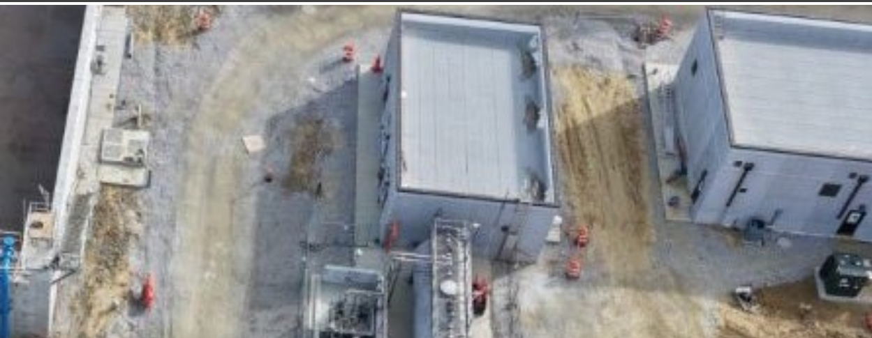
Fully commissioned Methanol facility
