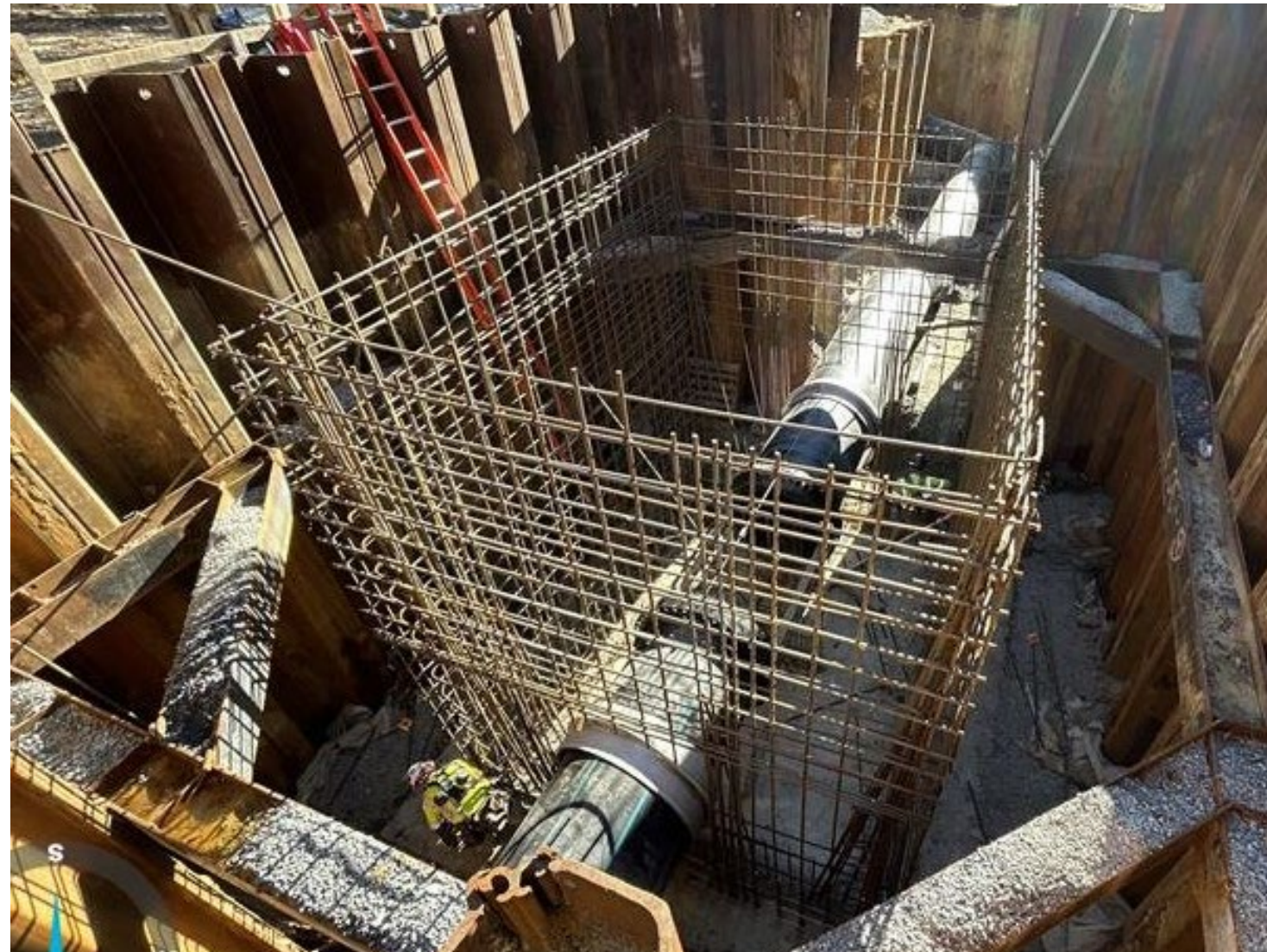
Instrumentation vault concrete
