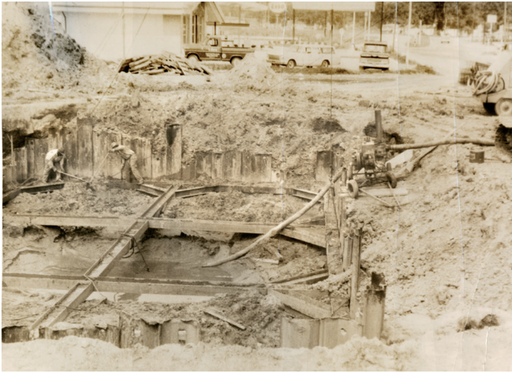
The HRSD network, which included 42 pump stations in 1966, continued to grow with the addition of facilities such as the Newtown Road Pump Station, photographed during construction in 1968.
