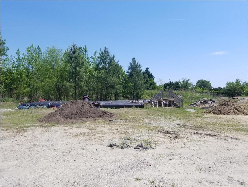
Miscellaneous materials, soil, and debris present in the JRTP storage area.
