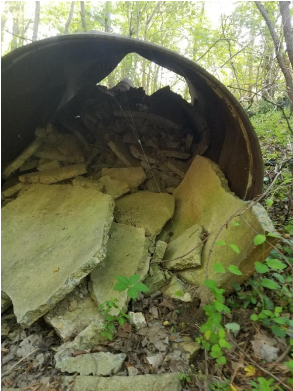
Debris along slope northwest of the JRTP sites.
