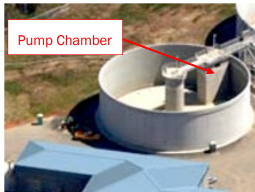
Figure 4-15. Tank with additional chamber for drain pumps
