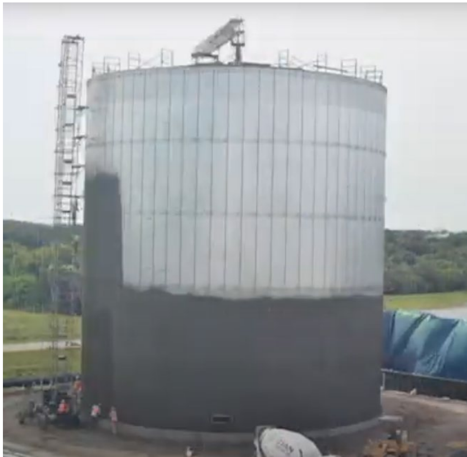
Figure 4-18. Prestressed Concrete Tank Construction
