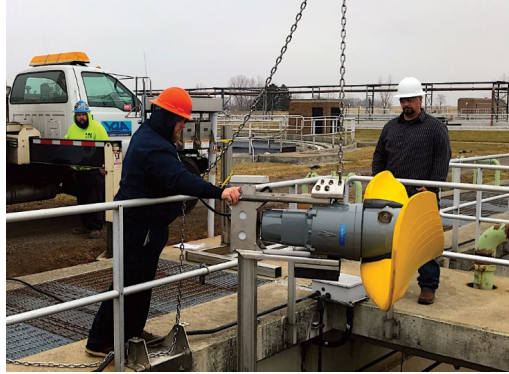
Figure 4-29. Mast-mounted submersible mixer
