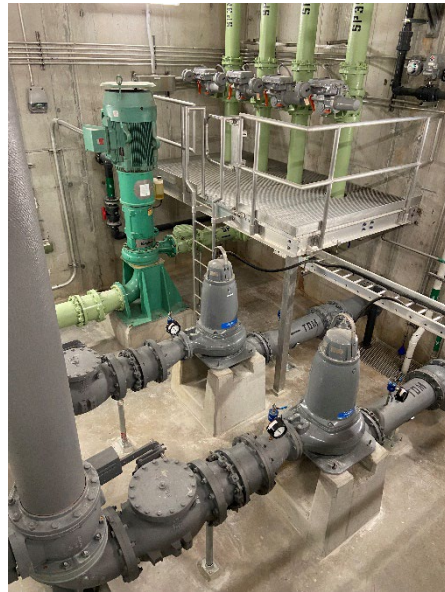
Figure 4-6. Dry Pit Submersible Pumps Installed at Woodstock OLSF
