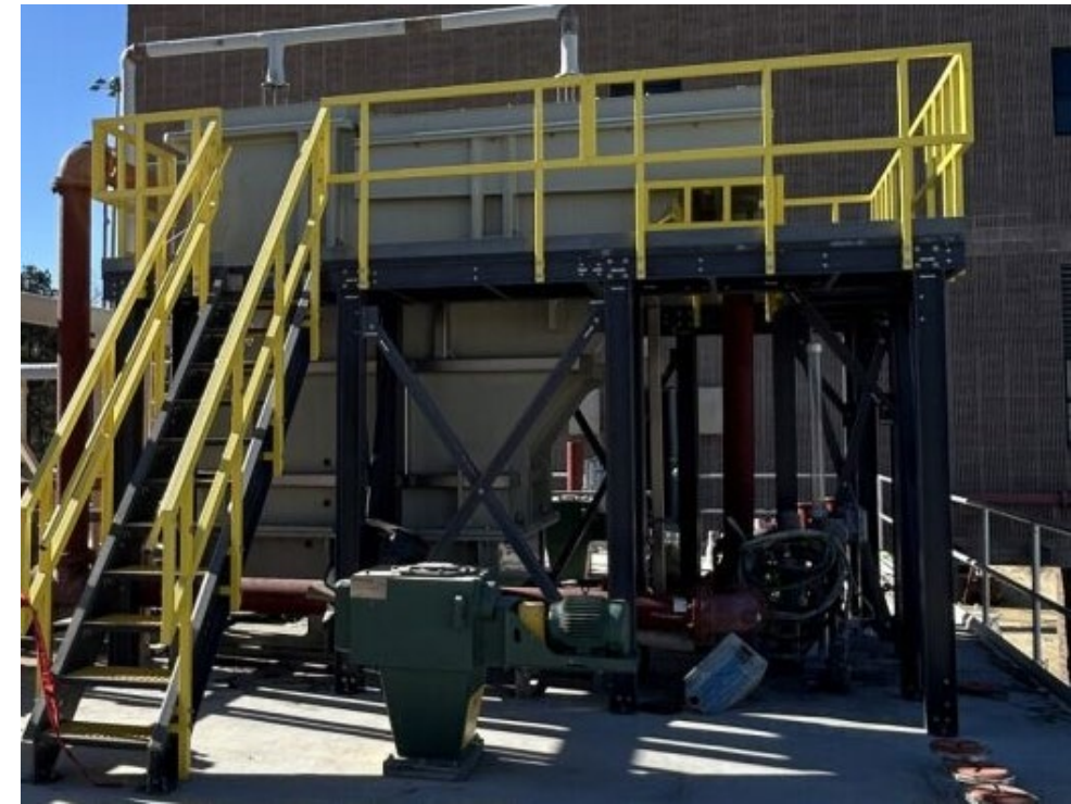
Blowers located in the Pre-Dewatering Building
