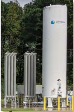
Liquid Oxygen Storage and Vaporizers
